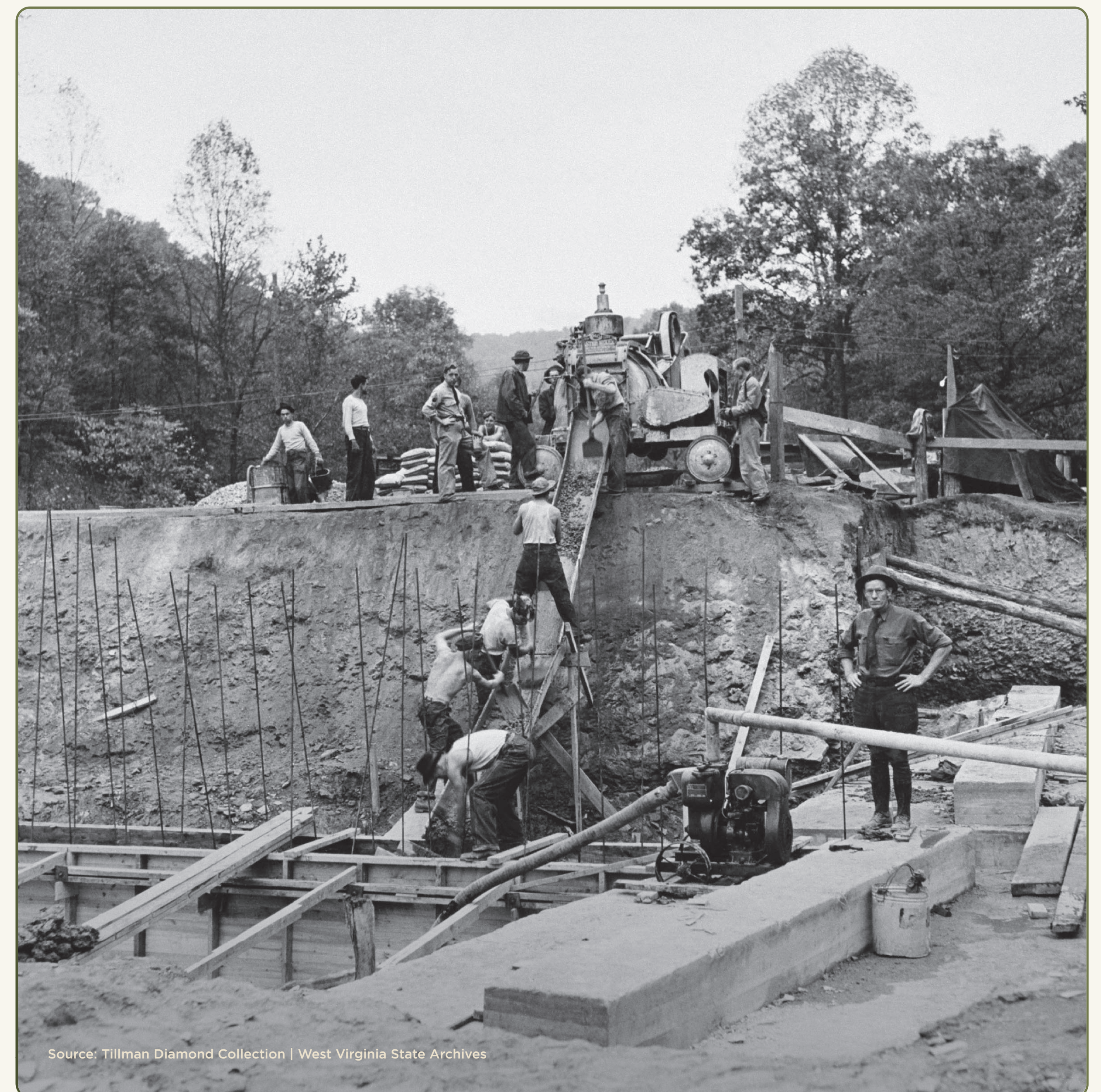
L.E.M. Foreman Walter Trail directs junior enrollees pouring concrete.
