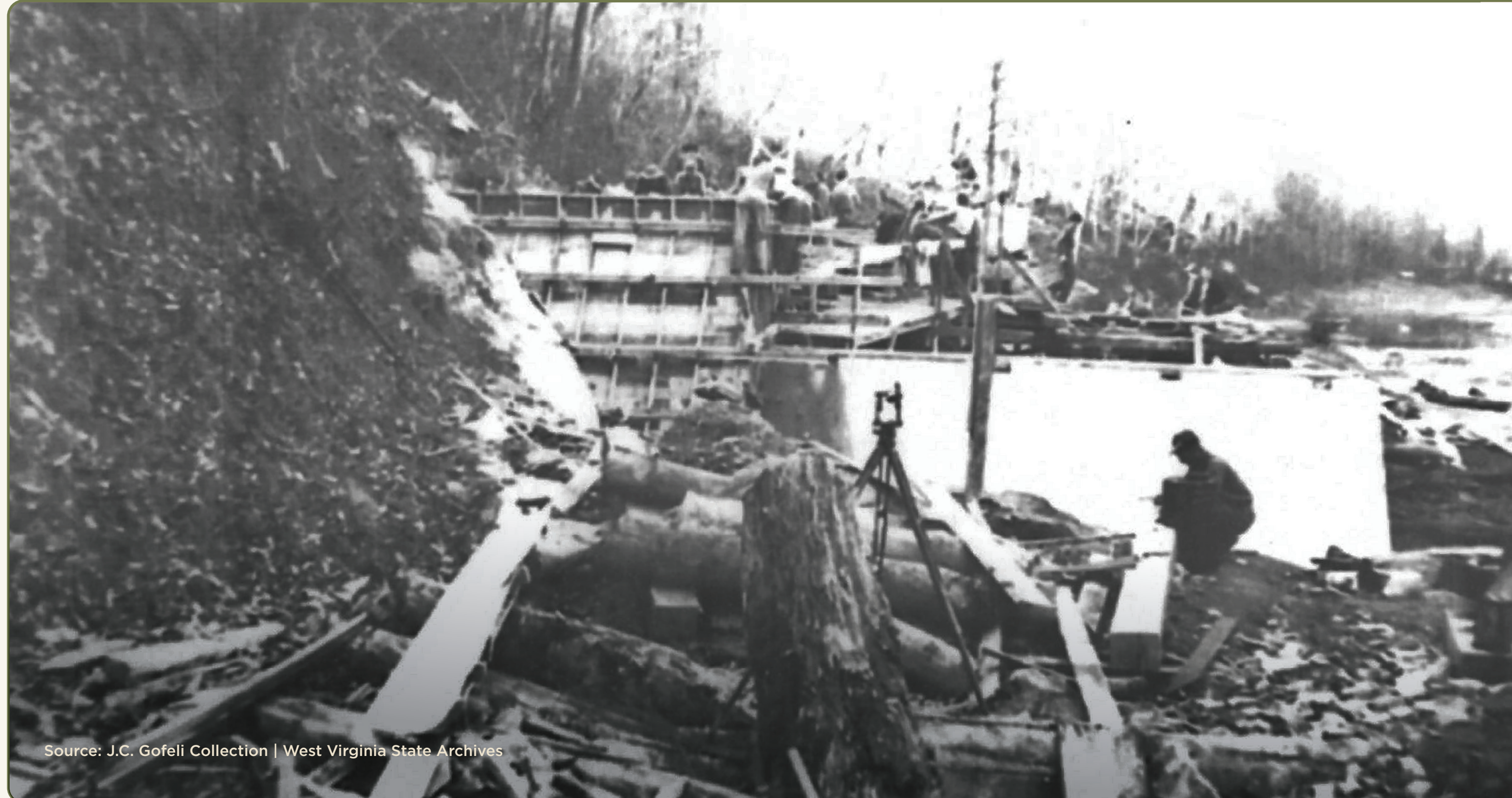
Construction of right abutment of dam.
