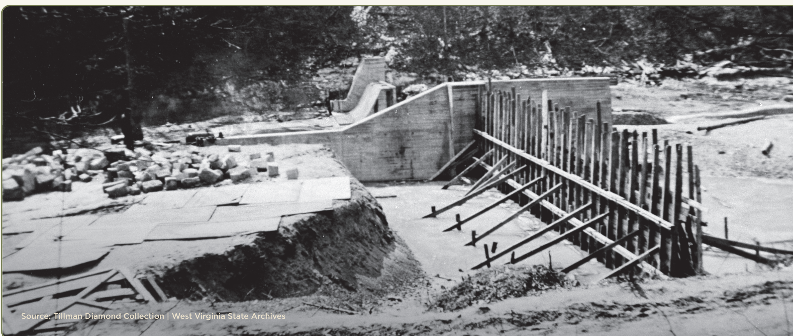
Construction of left anchor on left abutment of dam.
